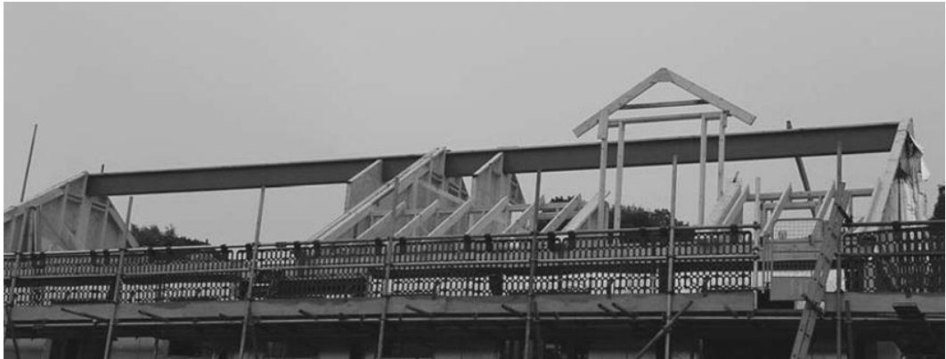
Photograph of a steel ridge beam.
